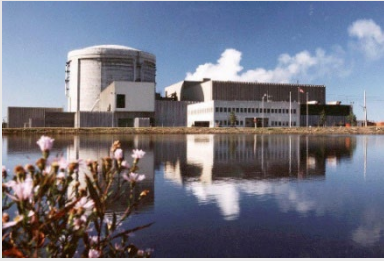
Neutron beams were critical to explain, and prevent downtime from, cracking issues at Canada's fleet of nuclear power reactors.
